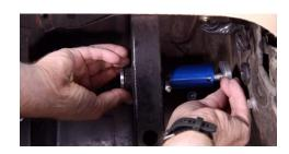
9. Install the steel flat washer onto the threaded rod.
