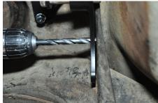
Go to the other side of the car and drill one hole and install a bolt. After you have a positively located the cross member drill the remaining holes.
